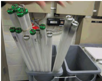
Audit: Spent lamps not properly stored.
