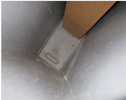
Follow-Up Visit: Broken lamp properly cleaned up.
